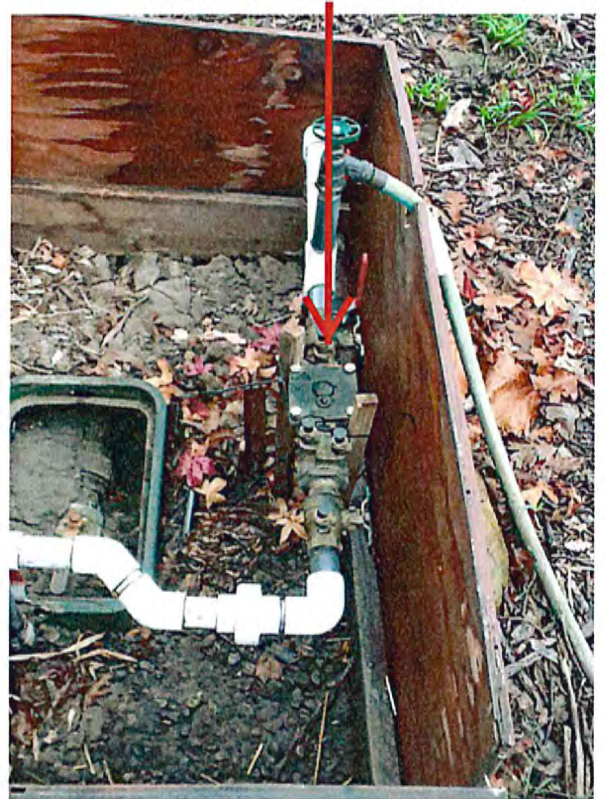
Irrigation RP Check Valve
