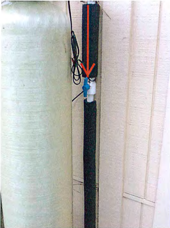
Caretaker Unit Shut Off Valve
