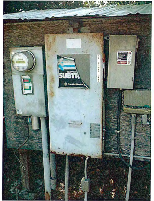
Well Pump Control Panel
