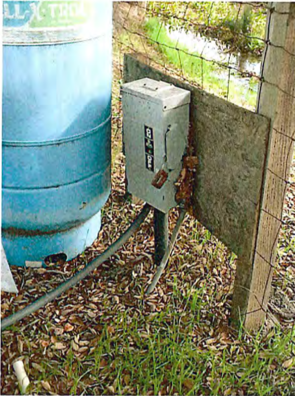
Pond Pump Disconnect
