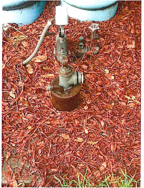
Old Well (not tested or inspected)
